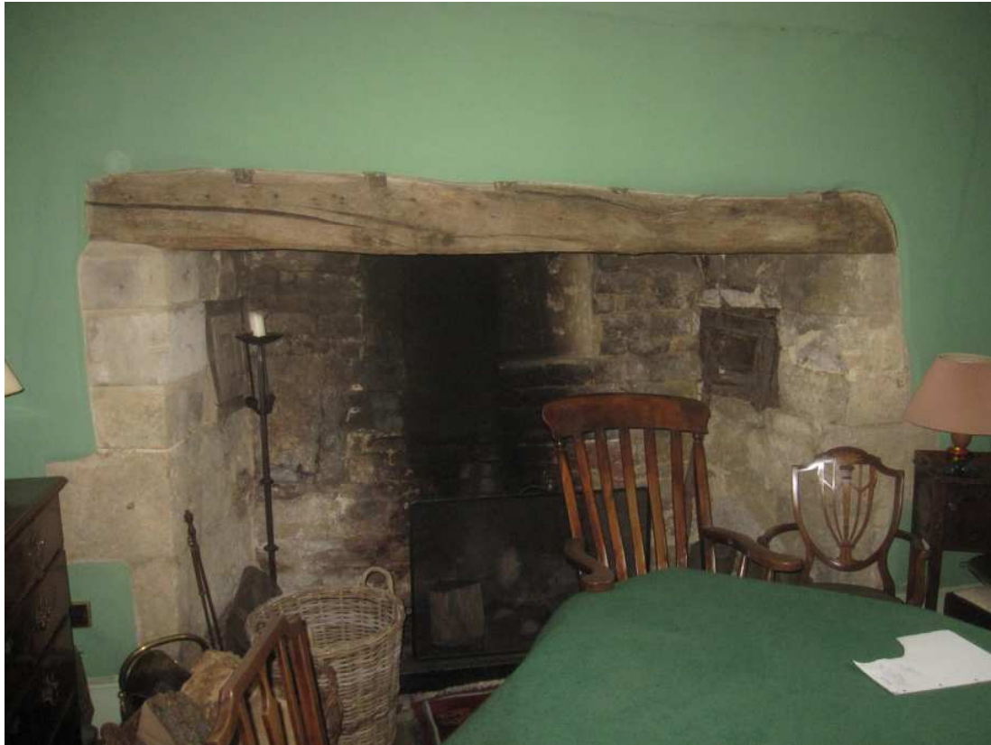
Fireplace to dining room (central room of main block, with recently inserted beam)
