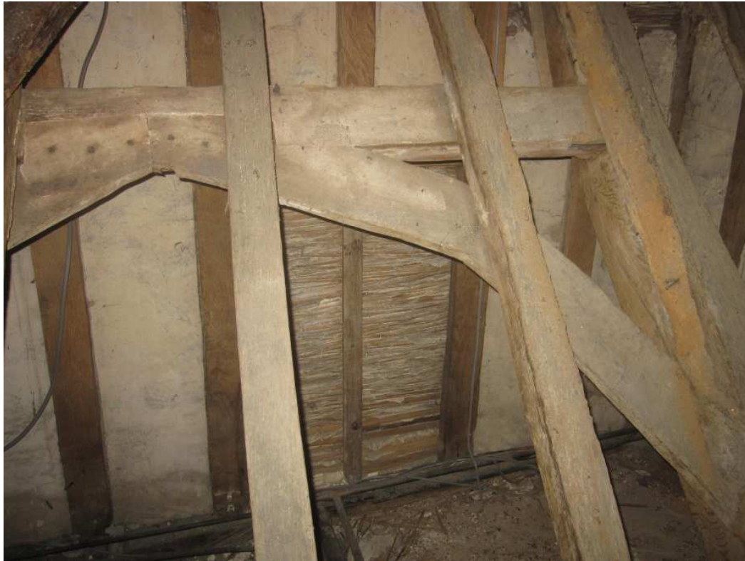
Bay T5/T6 (dated 1586-1611) from north, with cranked and nailed wind-braces
