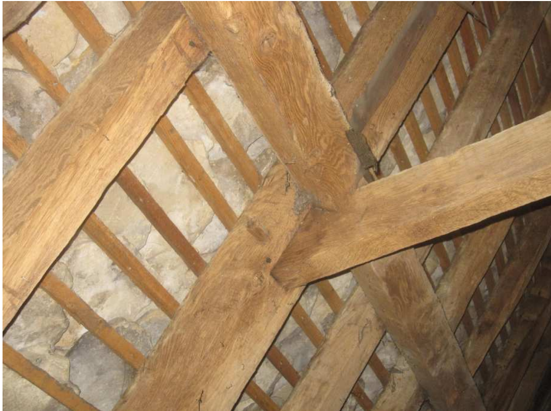
East face of roof truss T1 (dated 1678) to west end of main block, with carpenter's mark 'I'.
