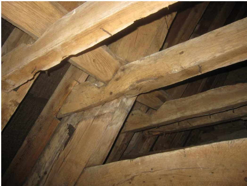
West face of truss T4 (dated 1586-1611) with tenoned purlin and lapped, nailed ceiling joists
